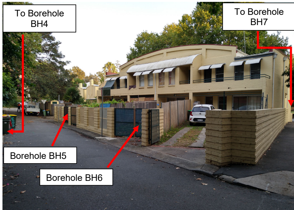
Photograph 10 – View west along Park Lane. The approximate positions of Boreholes BH4 to BH7 are indicated as shown.
