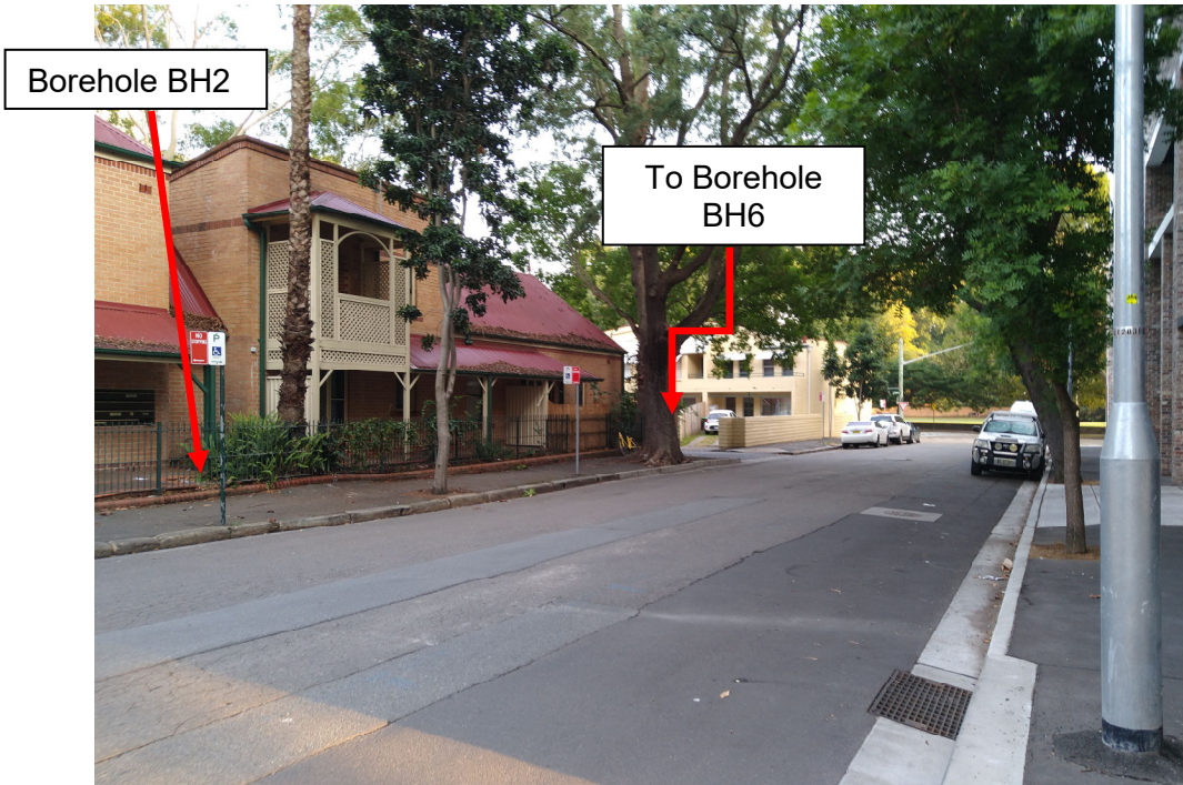
Photograph 5 – View north-west across Cowper Street. The approximate position of Boreholes BH2 and BH6 are indicated as shown.
